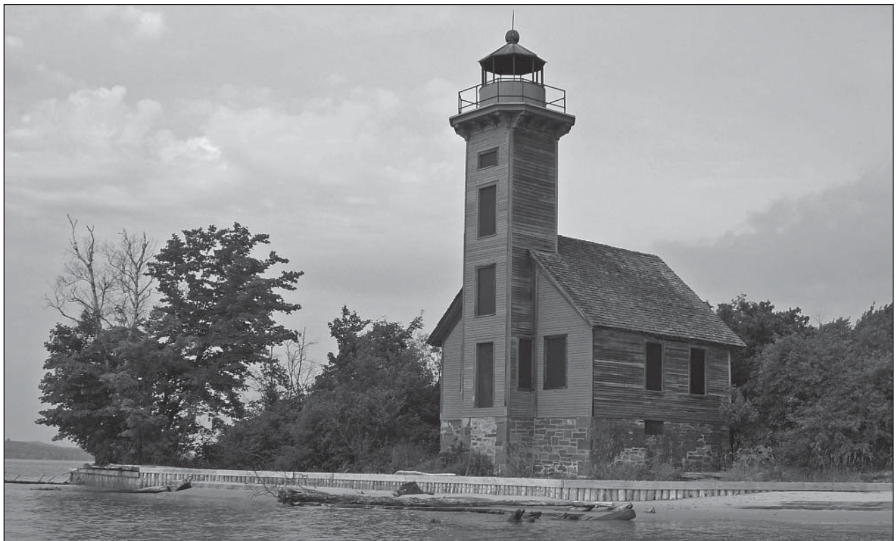
Grand Island East Channel Light from the northeast, July 2005. Salvaged original siding was reused on the north side of the building, which accounts for the difference in appearance.
