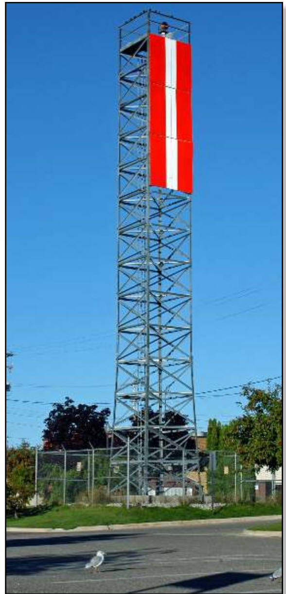
The skeletal rear range light tower
