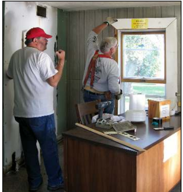
Tearing out ugly 1980's paneling in the new gift shop
