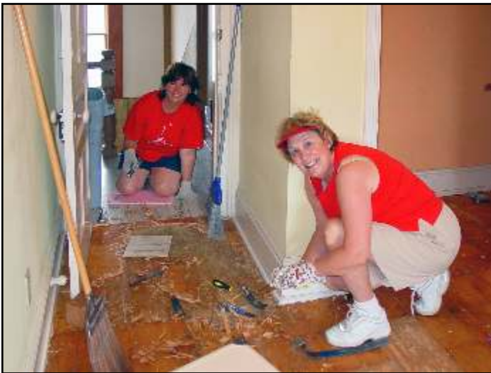
Removing thousands of nails from plywood on 2 nd floor
