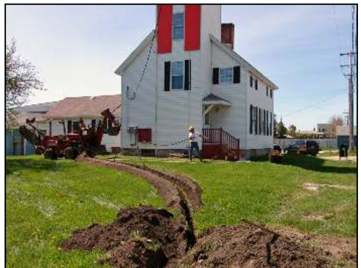
Moving the overhead electrical supply line to an in ground trench
