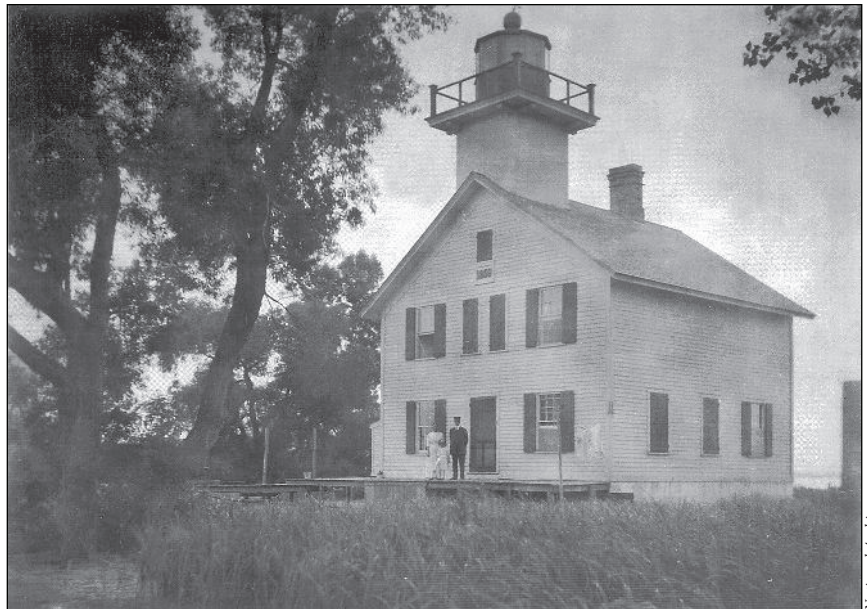
Front view of the timber-frame second Tail Point Light taken in July of 1913
